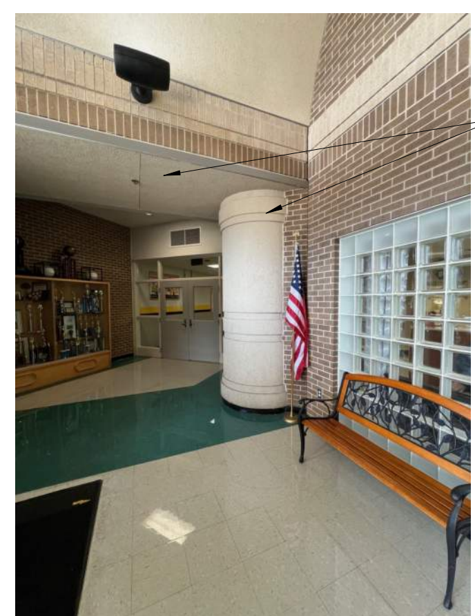
TYPICAL COLUMN IN LOBBY
