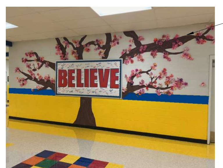
PAINT OVER EXISTING TREE- APPLY TYPICAL CORRIDOR PAINT - REFER TO SHEET 2/A7.1 FOR TYPICAL CORRIDOR PAINT
